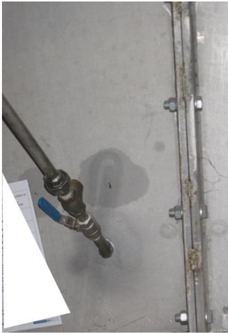
Picture: Direct dosage of enzyme into the pulper (no enzyme exposure). Courtesy of Buckman
